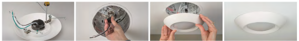
Step 1: Install torsion springs to the SMD6 trimbox
